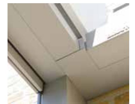
Waterafvoer via goot direct in steunpaal
